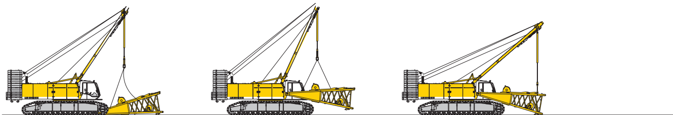
Unloading and assembly of boom foot
